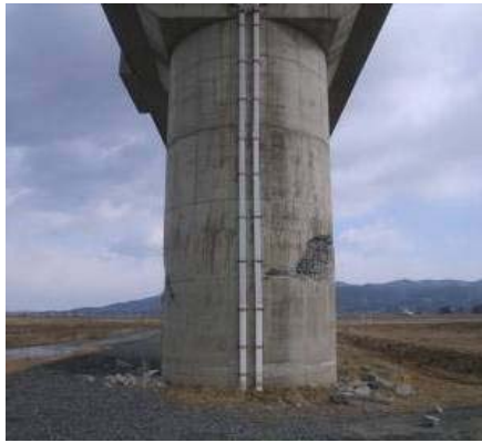
Photo 3 Damaged column
