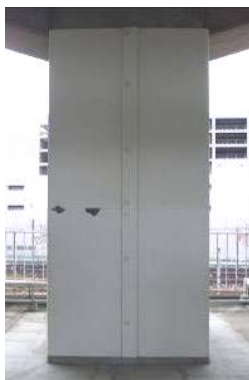
Photo 5 Seismic reinforcement using steel casing sections (interlocking joints)
