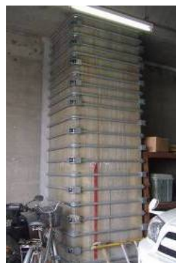
Photo 6 RB seismic reinforcement
