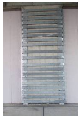
Photo 7 RP seismic reinforcement
