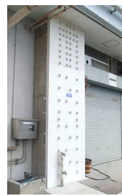
Photo 8 Single-face seismic reinforcement
