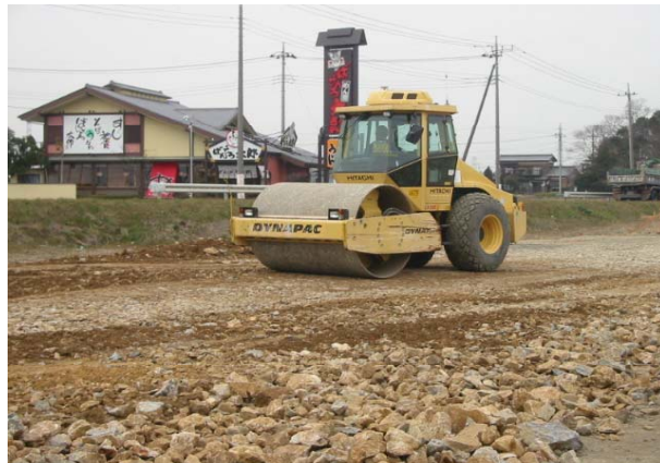
Fig. 3 Vibration Roller used in Pre-survey Study
