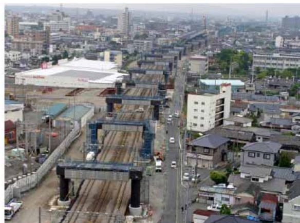
Condition prior to girder erection
