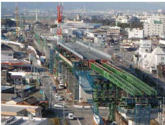
Girder launch yard in the direction of Hakata (by a municipal road)
