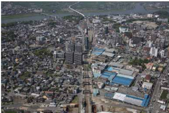
Urban facilities in the vicinity of the Bridge
