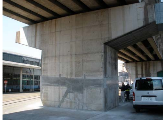
Hishida Viaduct P15
