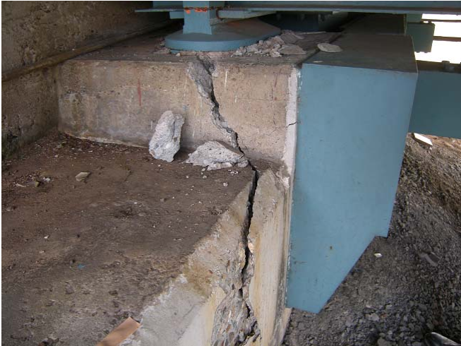
Tenjin Bridge A2 shoe
