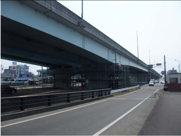
Kamedaohashi Bridge General view (Center left: P5 on up side; center right: P5 on down side)
