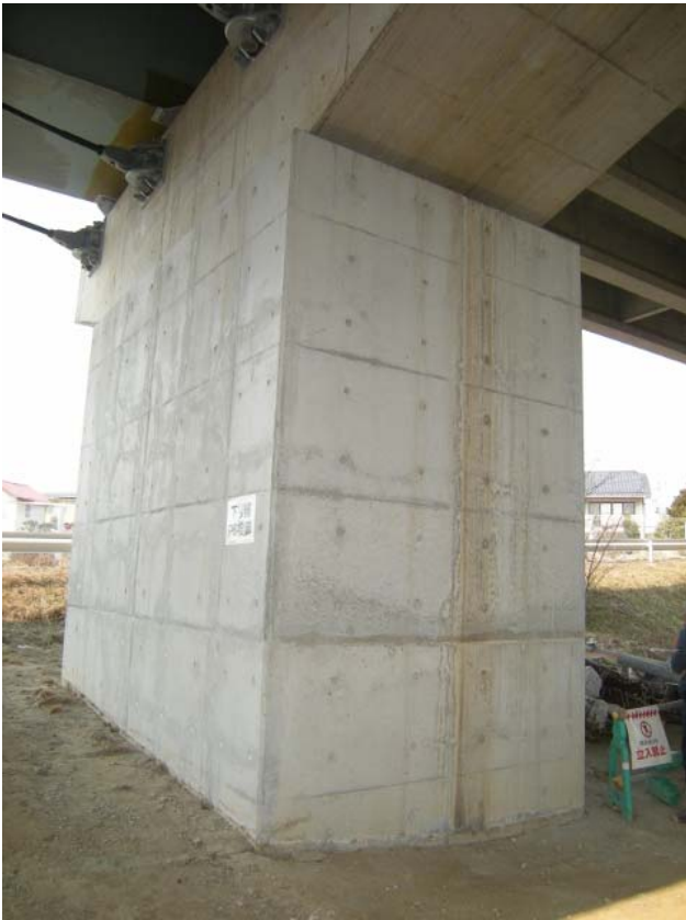
Kamedaohashi Bridge P6 No noticeable damage
