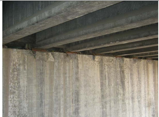
Daikokubashi Bridge P4 girder support
