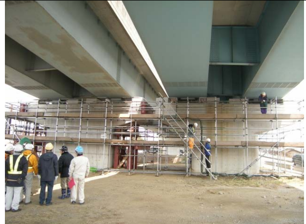
Kamedaohashi Bridge P5 (left: down side; right: up side)
