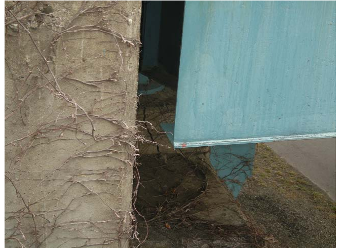
Tenjin Bridge A1 shoe
