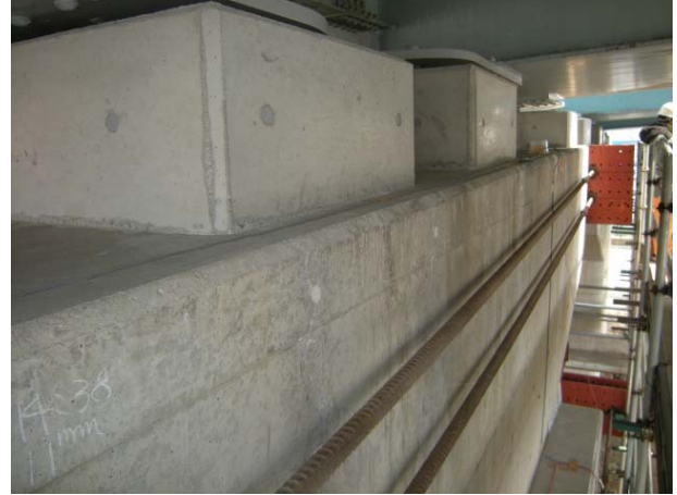
Kamedaohashi Bridge P5 on down side (stopper) Undamaged stopper
