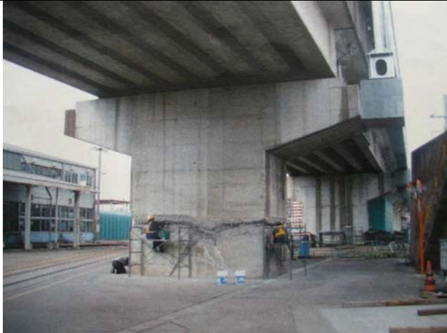
Hishida Viaduct P15
