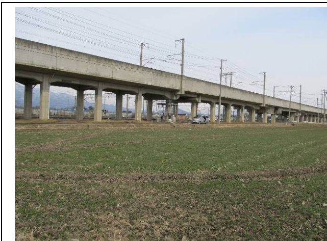
No. 1 Akabayashi BL R3 and subsequent rigid frames: undamaged
