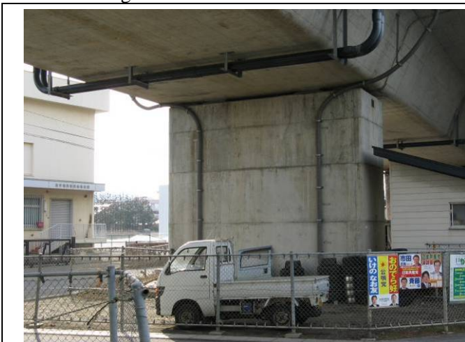
No. 2 Nishi Senboku BV Undamaged
