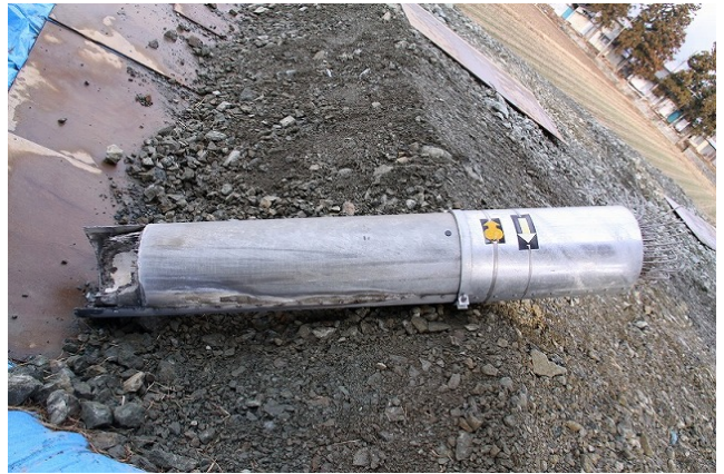
Broken catenary pole
