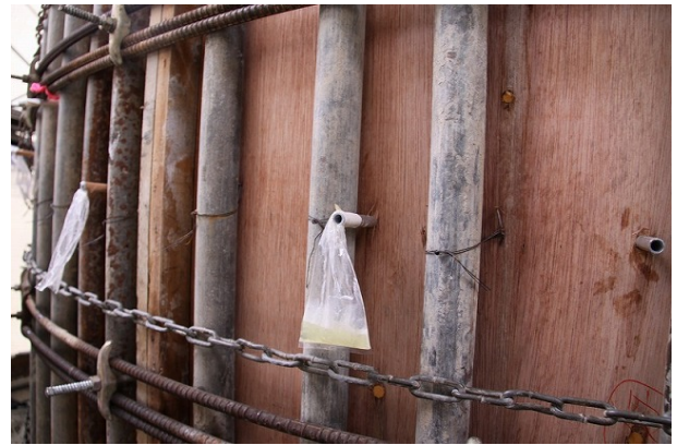
No. 1 Kitakamigawa Bridge
