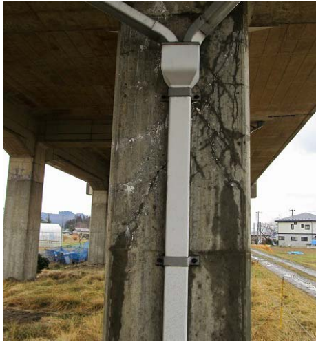
R3: The other side of the column shown above
