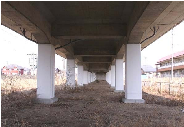
No. 3 Hizume BL R1 and R2: Undamaged Columns had already undergone seismic retrofitting with steel jacketing.
