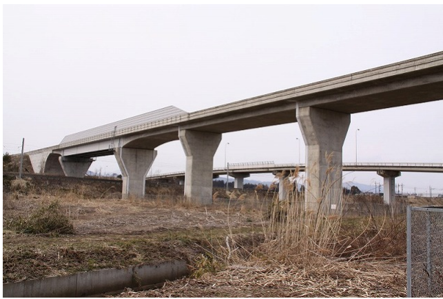
Miyanome Bridge on the Kamaishi Expressway Undamaged
