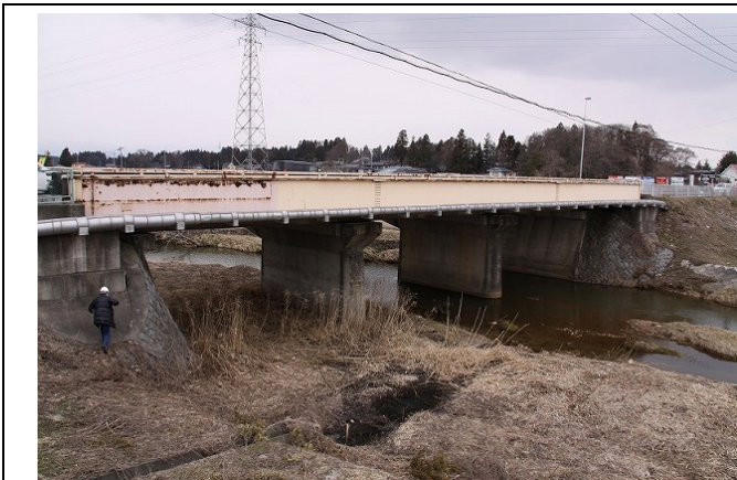
Iide Bridge on National Road No. 4
