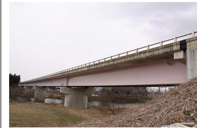
Kitakamigawa Bridge on the Kamaishi Expressway Twin main-girders PRC slab: undamaged
