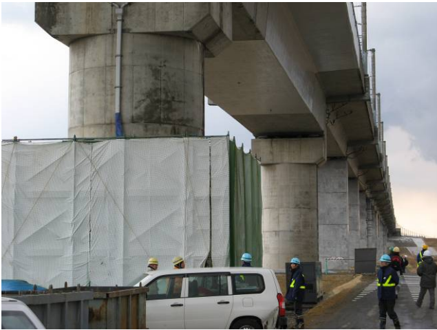
No. 1 Kitakamigawa Bridge
