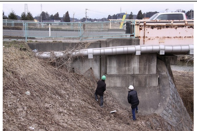
Iide Bridge on National Road No. 4
