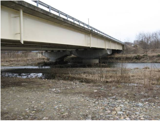
Toyosawagawa Bridge on the Tohoku Expressway: undamaged
