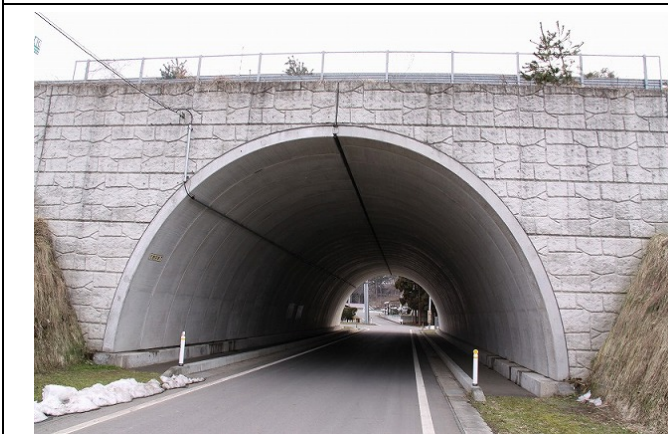
Precast three-hinge tunnel (Near Miyanome Bridge on the Kamaishi Expressway): undamaged
