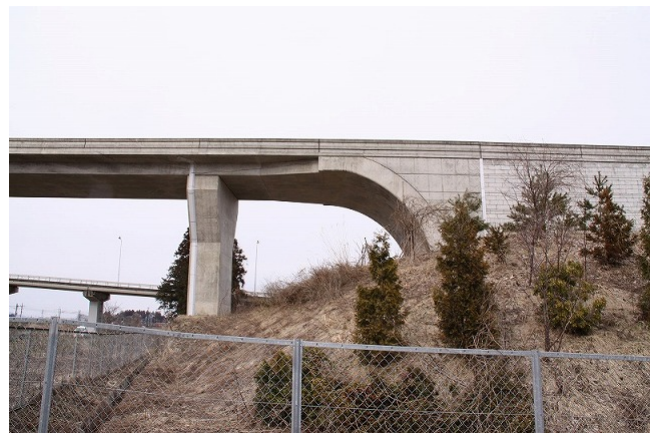
Miyanome Bridge on the Kamaishi Expressway Girder end is integrated with abutment. Light fill is used at the back of the abutment
