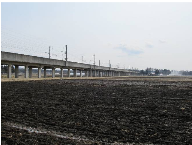
No. 5 Inohana BL R1 to R12 (Not yet seismically retrofitted)
