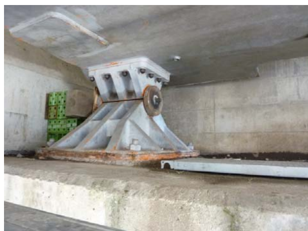
Fig. 3 Bearing after repair
