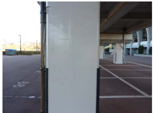
Fig. 4 Shear cracking in column of rigid frame viaduct
