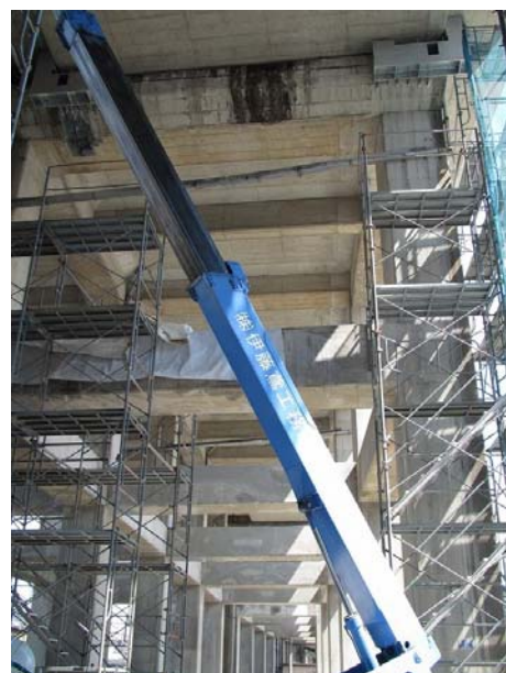
Fig. 2 Beams after repair and steel shear stopper being installed
