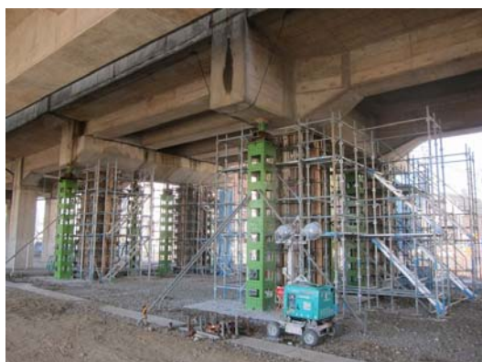
Fig. 2 Emergency repair work
