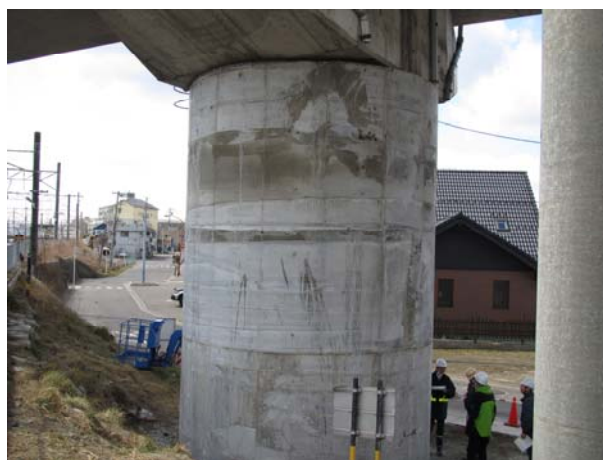
Fig. 2 Repaired bridge pier of Iwakiri viaduct
