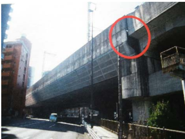
Fig. 1 General view of the bridge (Source: East Japan Railway Company)
