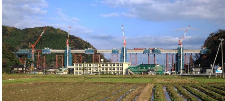
Photo 1 cantilever method of girders erection
