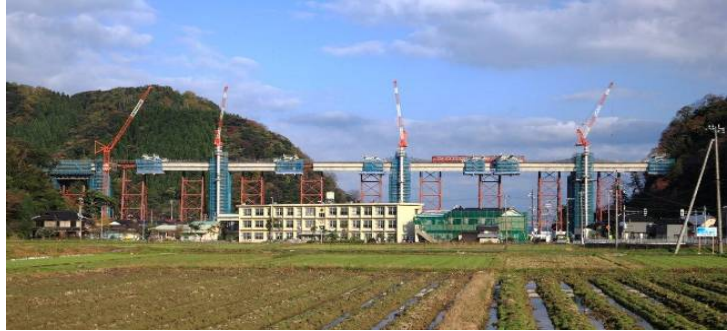
Photo 1 cantilever method of girders erection
