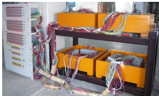
Picture 1 Overview of macro-cell corrosion measurement
