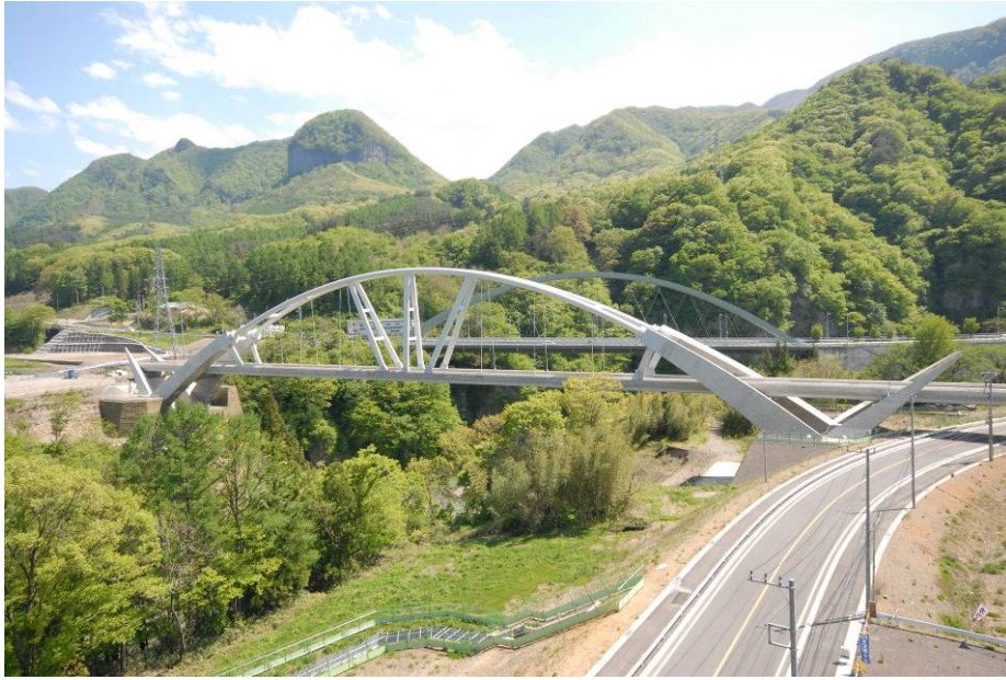
The 3rd Agatsuma River Bridge
