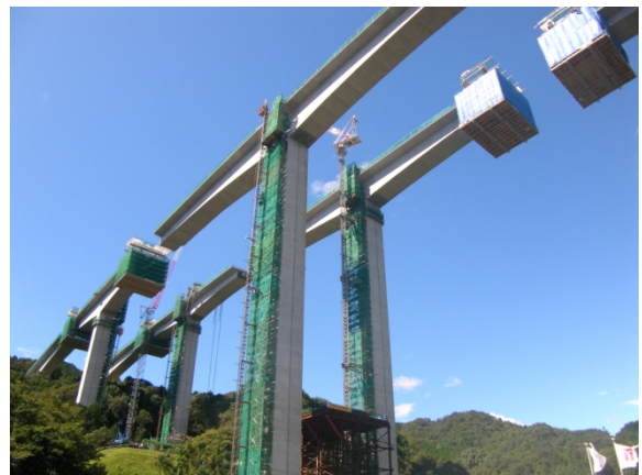
Fig. 6 Segmental construction of balanced cantilever girder
