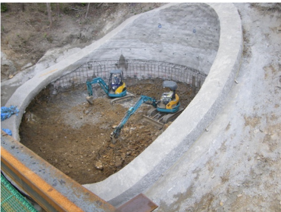
Fig. 7 Cut bamboo shaped landslide-prevention wall
