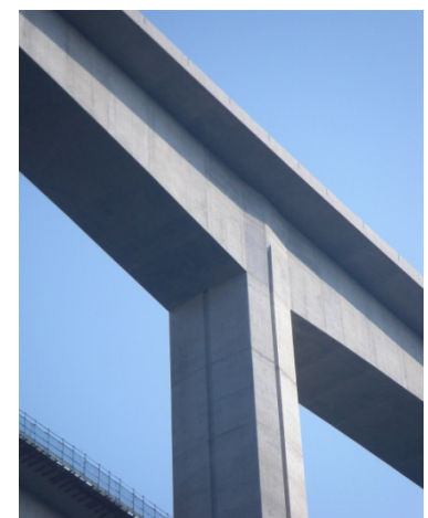
Fig. 4 The eight-faced piers
