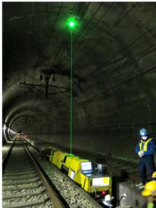
Fig. 7. Device in operation in tunnel's central passage
