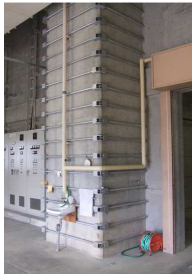
Photo 4. Column with a partitioning wall
