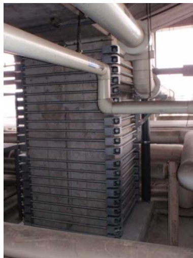
Photo 8. RC column in an occupied area and surrounded by obstacles
