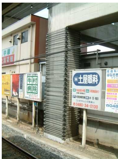
Photo 6. Column in a narrow space near a railway track
