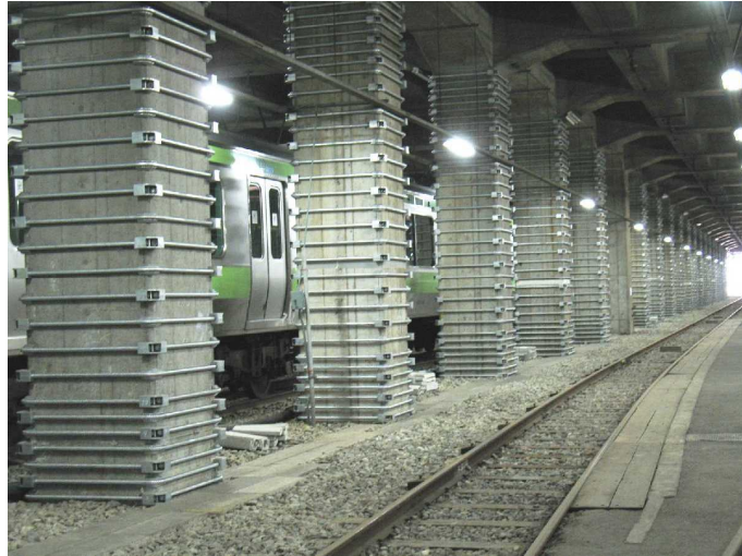
Photo 7. Columns in a narrow space near a railway track
