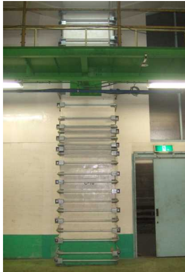
Photo 5. Column with an attached bracket
