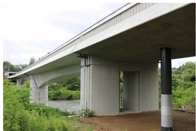
Figure 7. Wide overhang for the open channel
