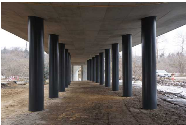
Figure 6. The shape of the Nishikoen Viaduct
