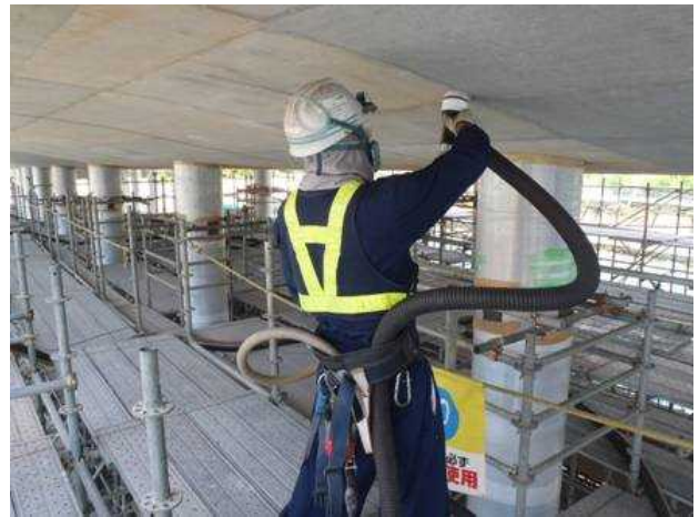
Figure 10. Polishing by sandblasting
