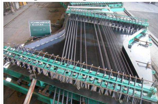
Figure.7. Arrangement of prestressing
