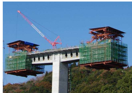
Figure 9. Cantilever construction
