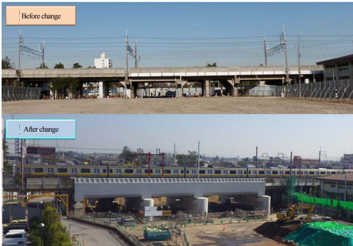
Fig. 13 View when completed (when underpinning is completed)
