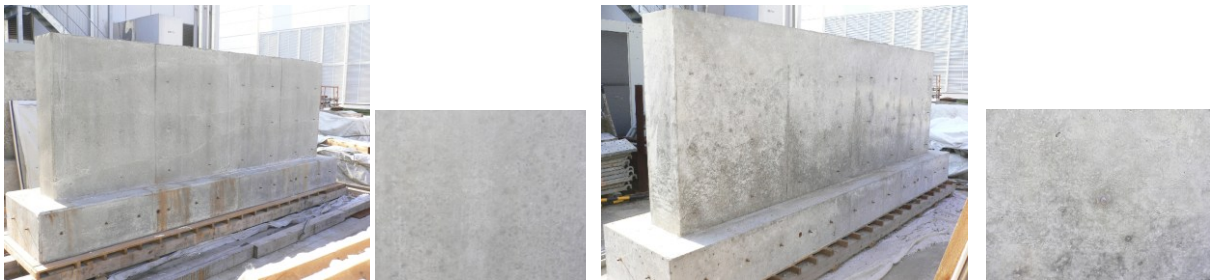
(1) Continuous drainage and moist curing
