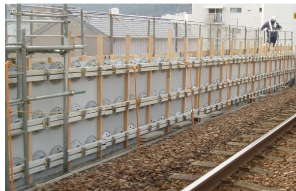
Photo 6. Railway side wall (working near railway traffic)
