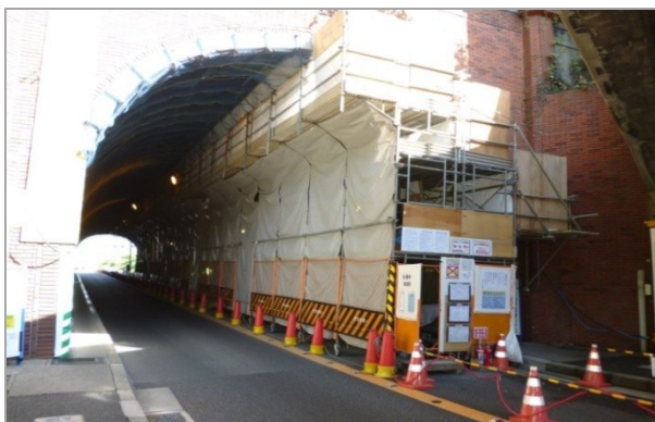
Photo 5. Tunnel lining (one-way alternate traffic)
