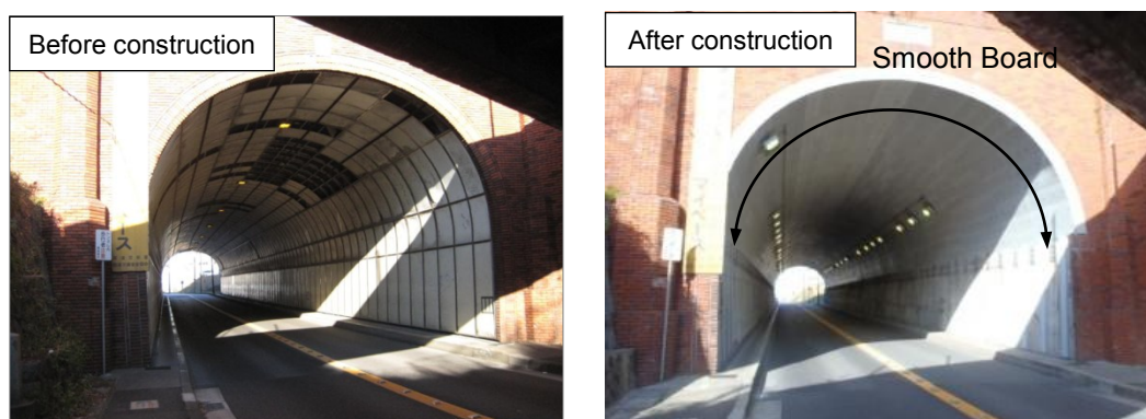
Photo 9. Repair of tunnel lining (additional concrete cast to increase the thickness)
