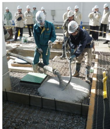
Photograph 5 Construction using a pump
