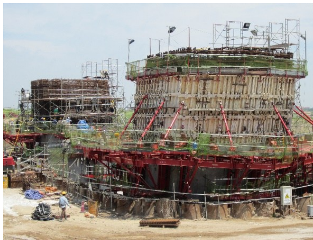
Photo 4. Installation of self-climbing work floor
