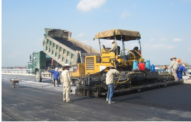
Photo 9. Construction of pavement
