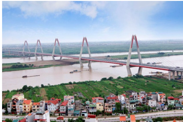
Photo 1. General view of the Nhat Tan Bridge
