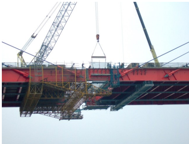
Photo 8. Closing of main girders
