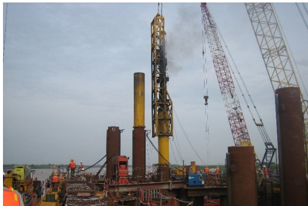
Photo 3. Final driving using diesel hammers
