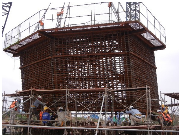
Photo 5. Erection of prefabricated steel cage
