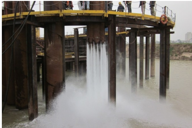
Photo 2. Vibro-method combined with water jet
