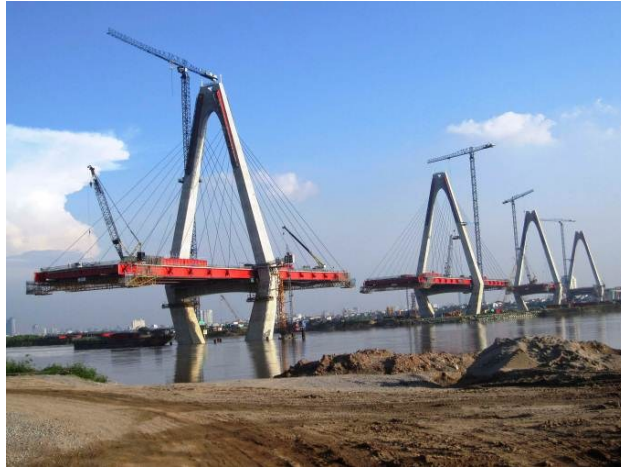
Photo 7. Erection by means of balancing cantilever erection method
