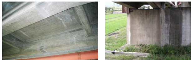
Photo 2. Superstructure and substructure before renovation
