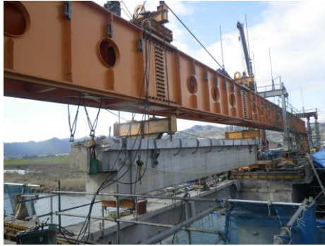
Photo 4. Removal of Gerber girders
