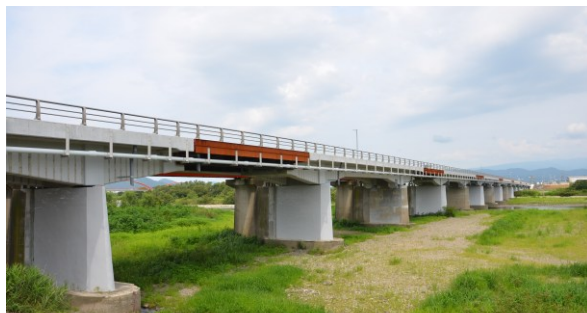
Photo 8. Renovated Genta Bridge
