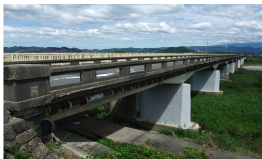
Photo 1. Genta Bridge before renovation
