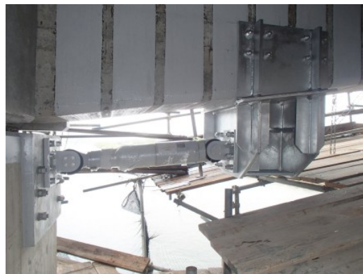
Photo 7. Installation of damper
