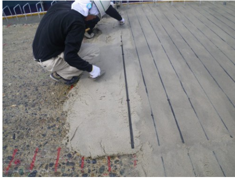
Photo 6. Reinforcement of upper surface of floor slab
