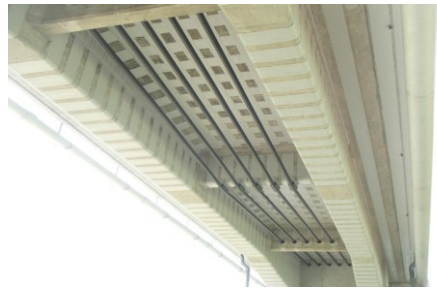
Photo 3. Reinforced section with external cables
