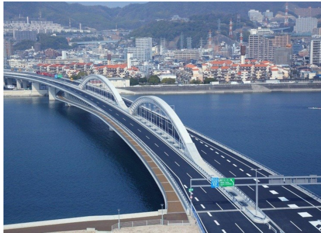
Photo 1. Ootagawa Bridge after completion
