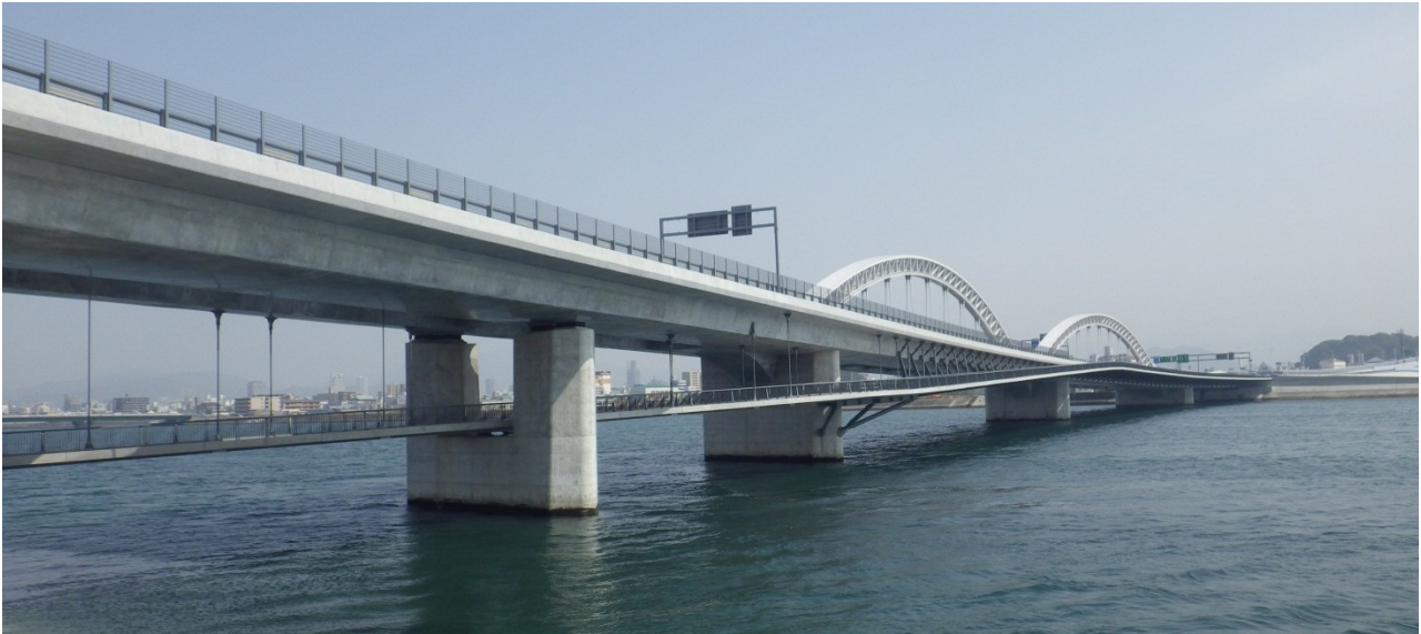
Photo 5. Ootagawa Bridge after completion
