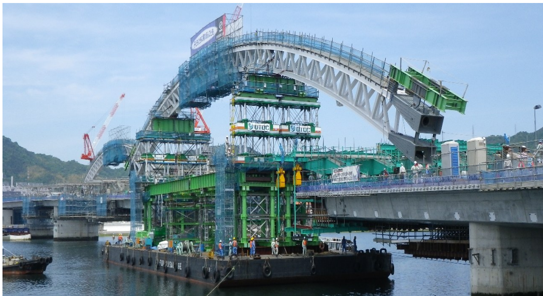
Photo 4. Simultaneous construction of the arch's main structures using a barge
