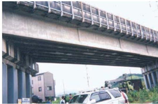
Fig. 4 Inspected PC girders
