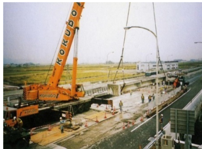
Photo 1 Removal of beam
