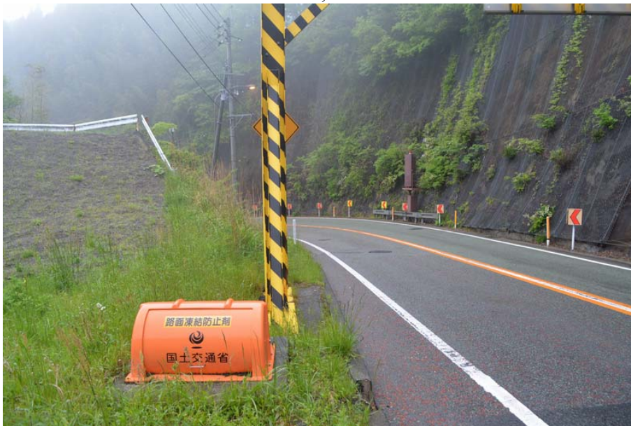
Photo 3 Surface antifreeze agent storage container
