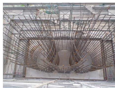
Figure 6 Reinforcement Arrangement of Pier
