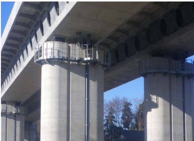
Figure 7 Drainage Pipe in Pier Slit
