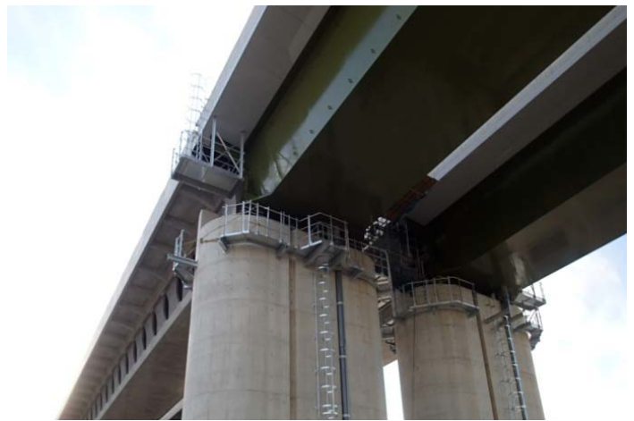
Figure 8 Joint Between PC Bridge and Steel Bridge
