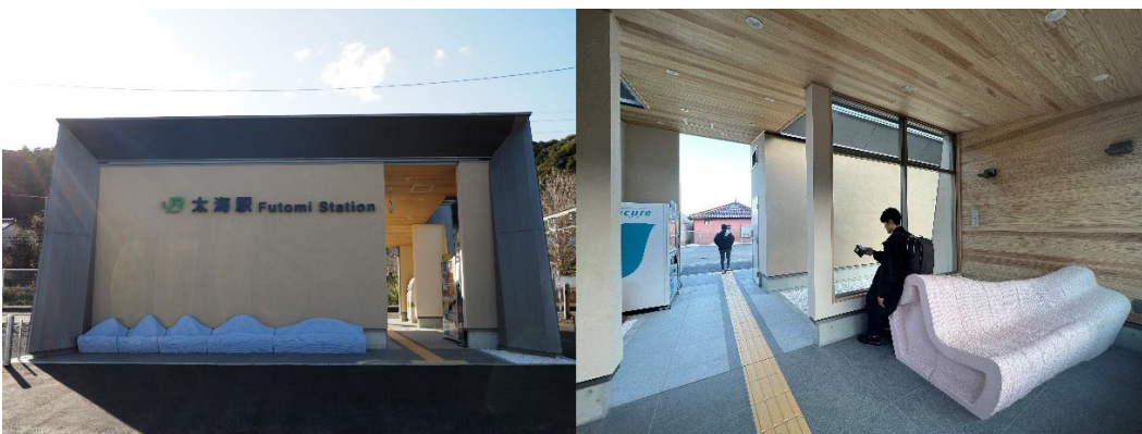
3DCP bench installed at Futomi Station
