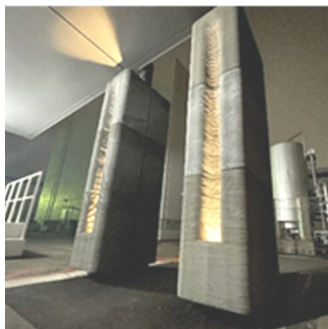
Photo 1: RC strut of roof with multi functions
