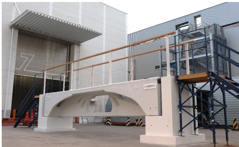
Photo 3: Pedestrian bridge utilizing topology optimization analysis and 3DCP
