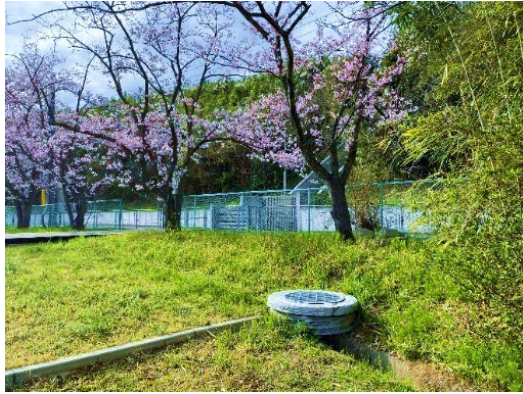
Fig.5 Installation of water catchment basin printed by 3DCP
