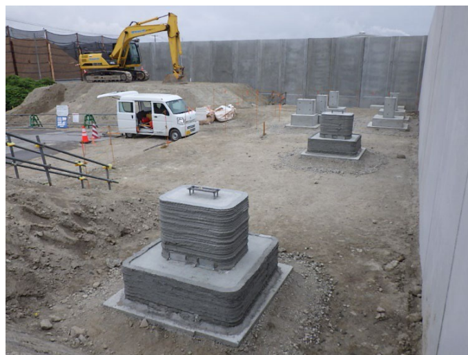
Example of Application: 3D Printed Foundation Formwork
