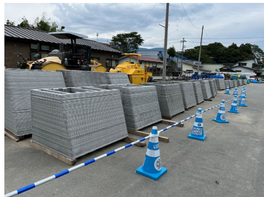
a) The prefabricated members
