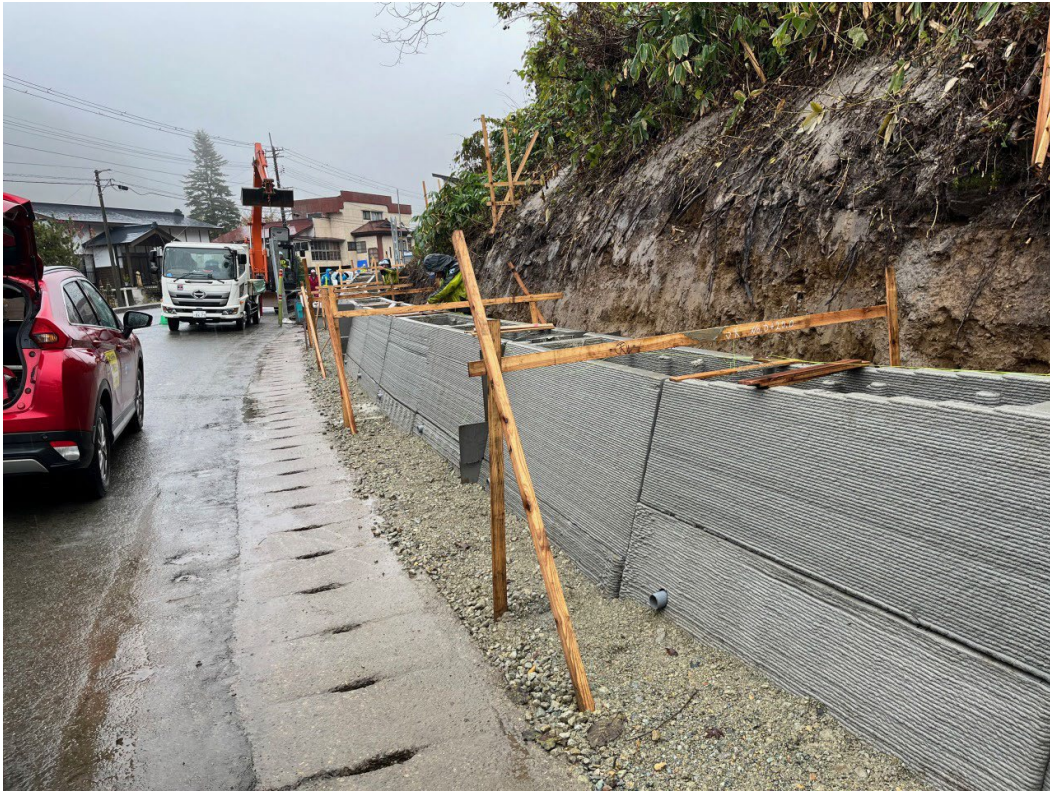
Fig. 3 Installation of the prefabricated formwork members
