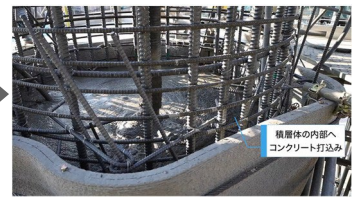
Concrete placement
