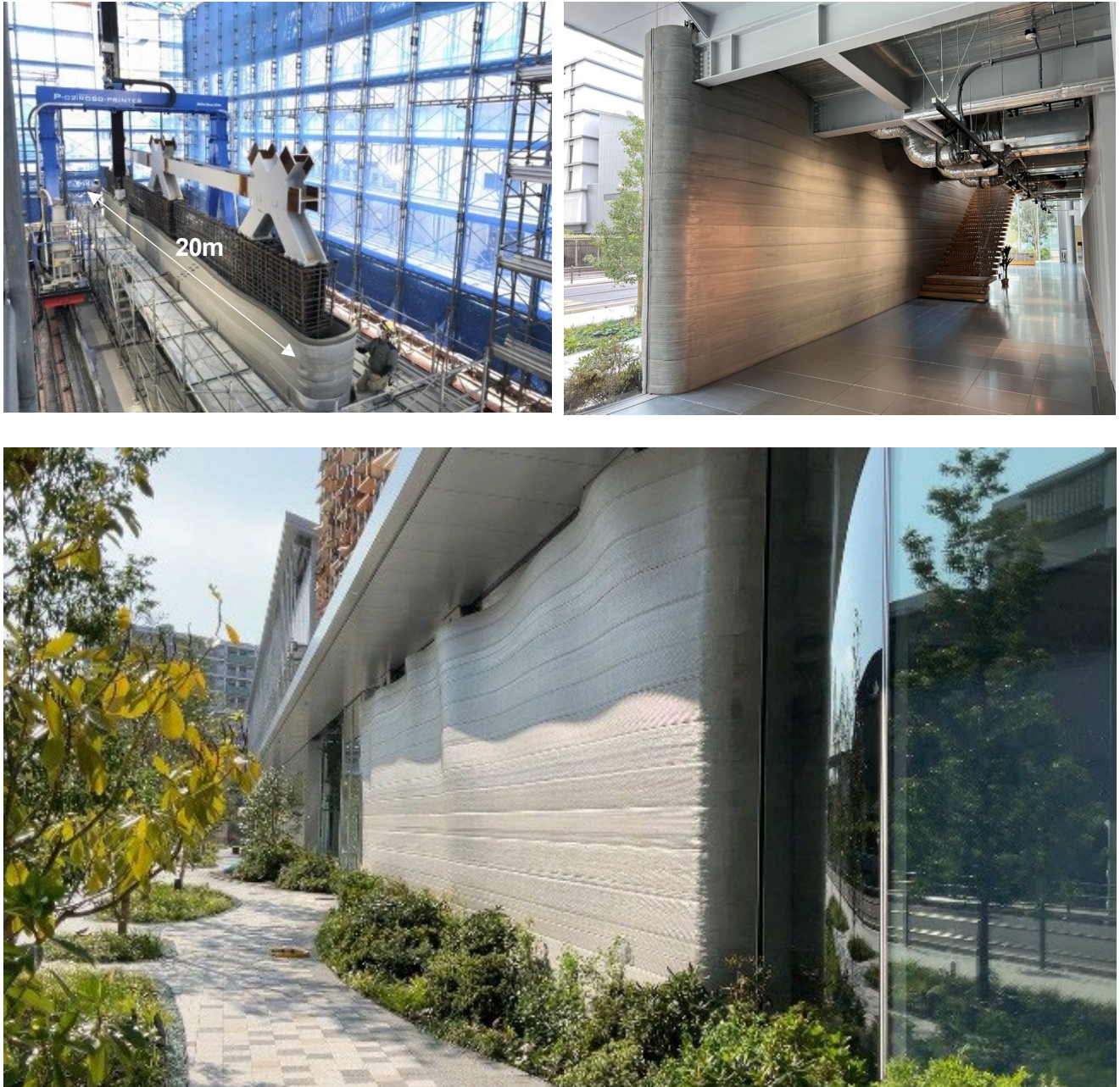
Fig. 7 Application at NOVARE
