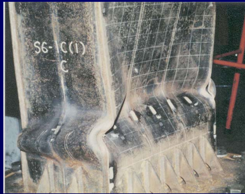
Box: Weak stiffeners
