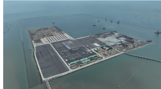
Photo 6: Patimban Port Construction in Sep, 2024
