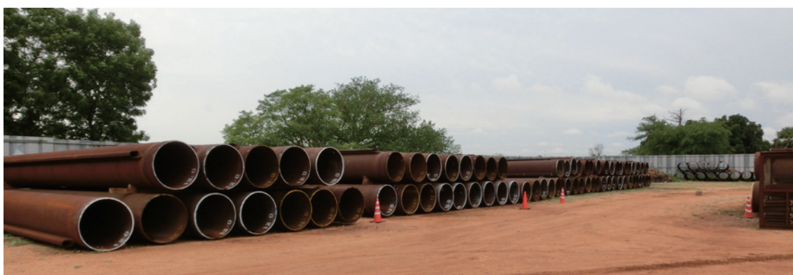
Photo 12: Steel Pipe Sheet Piles Exported from Vietnam
