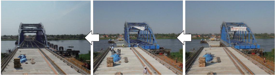
Photo 8: Lateral Sliding of Langer Bridge
