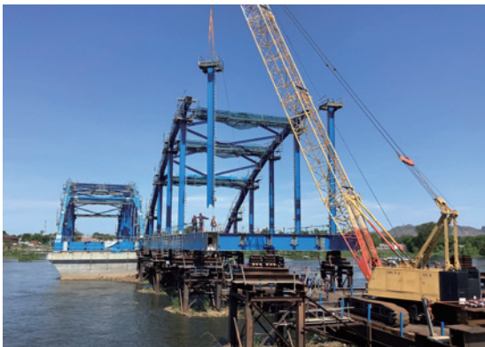
Photo 13: Erection of Langer Bridge on Temporary Bridge
