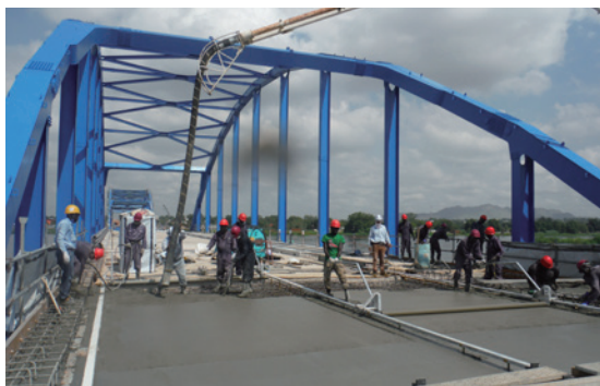
Photo 10: Bridge Slab Concrete Casting
