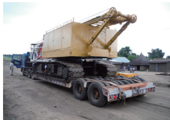
Photo 3: 1 st Cargo (80t Crane) Arrives at the Site
