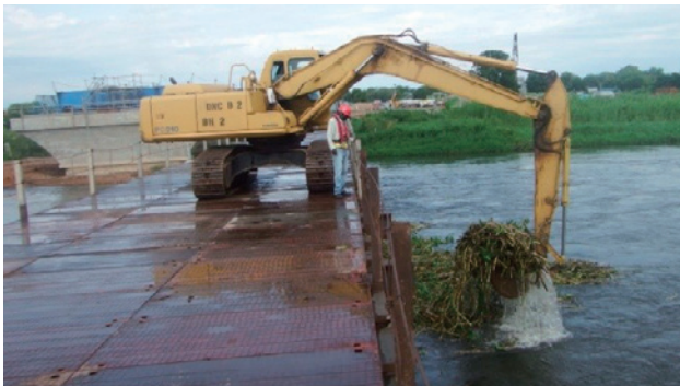
Photo 6: Site Maintenance by Local Staff
