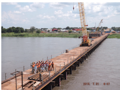
Photo 4: Temporary Bridge Completion
