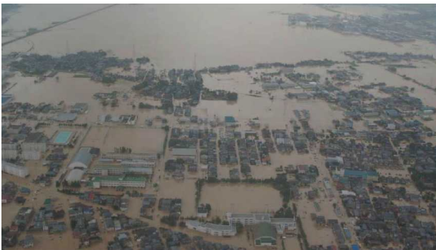
Photo 3 Flood-damaged Sanjo City
