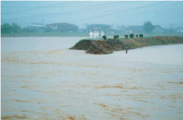
Photo 2 Broken dyke along Igarashi River (source: Sanjo City office)
